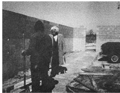
JOY OF HEAVEN BIBLE INSTITUTE EARLY STAGES OF CONSTRUCTION
