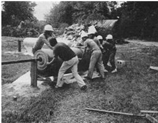
CONSTRUCTION WORKERS AT JOY OF HEAVEN BIBLE INSTITUTE
