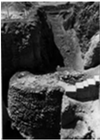
Figure 6.1. Stone watchtower unearthed at ancient Jericho. This tower dates to approximately 8000–7000 B.C.E. and was part of the walled fortifications of the city. It is one of the oldest human structures still standing. (Photograph by Mitchell G. Reddish)
